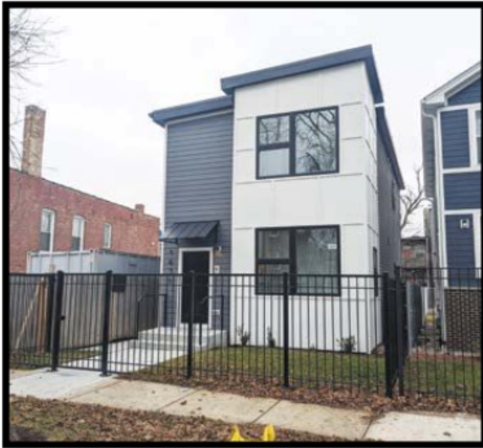
A modern modular home nearing completion.
